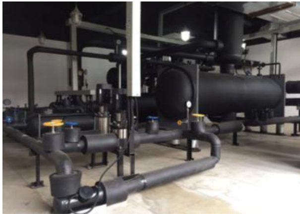
<New experimental converter of ocean thermal energy>
