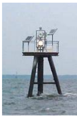
Battered pile dolphin
