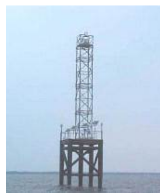
Multiple pile platform
