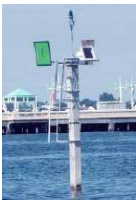
Single wood pile
