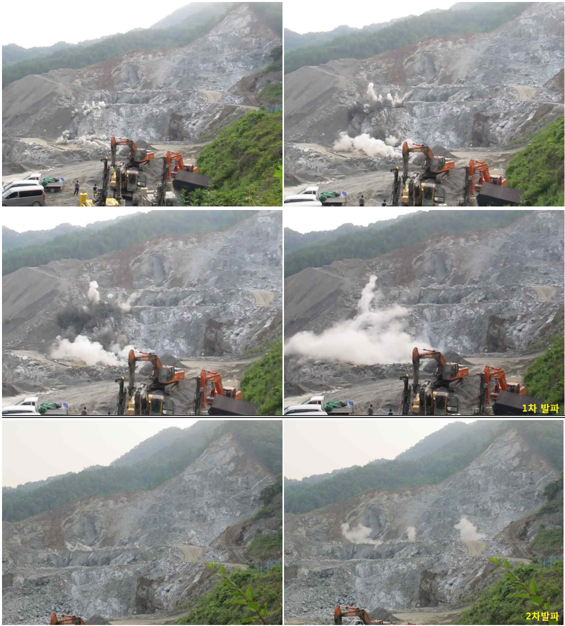
Figure 3.1.18 Blasting site in Hoengseong quarry.
