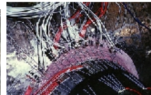
Hot spot region in a tubular joint, instrumented for strain measurements and crack growth monitoring by the potential drop method.
