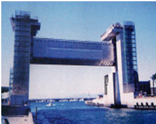
Fig. 10.2.64. Area C(left) - water gate at estuary, Area E(right) - floating flap barrier
