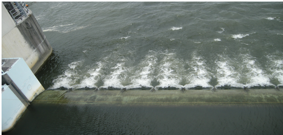
Fig. 10.1.19. Discharge water of overtopping through Sluice gate
