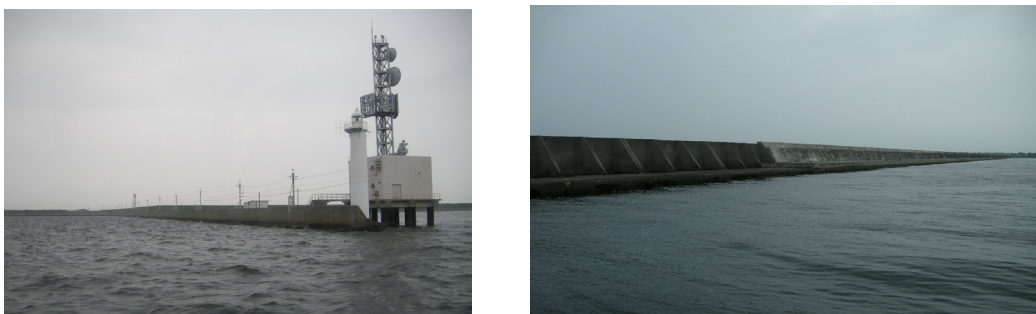
Fig. 10.1.18. Seawall at Nagoya port, Japan
