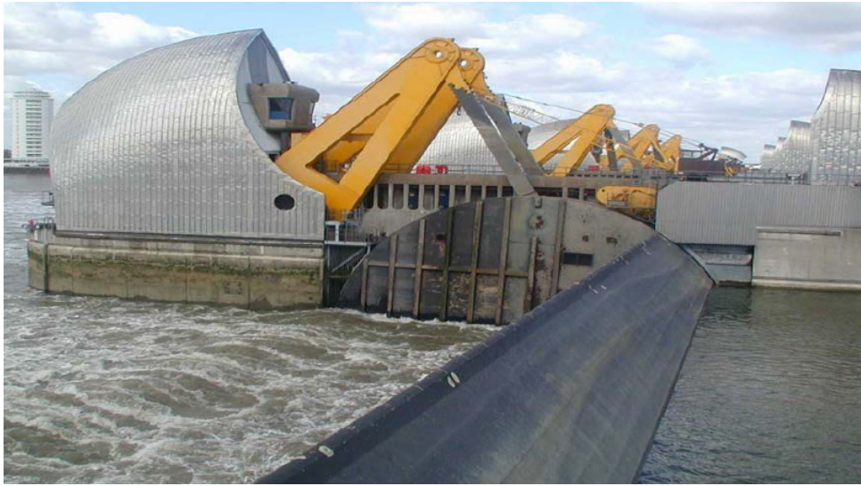
Fig. 10.1.32. Thames barrier at England
