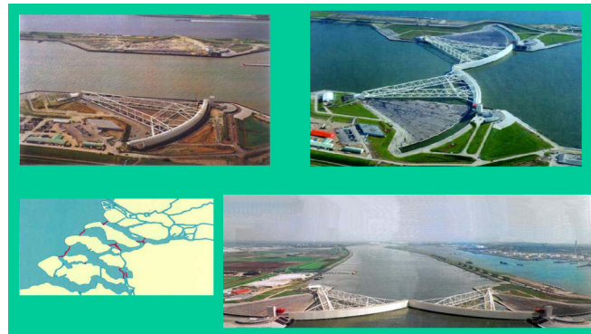
Fig. 10.1.30. Storm surge Sluice gate of Netherland
