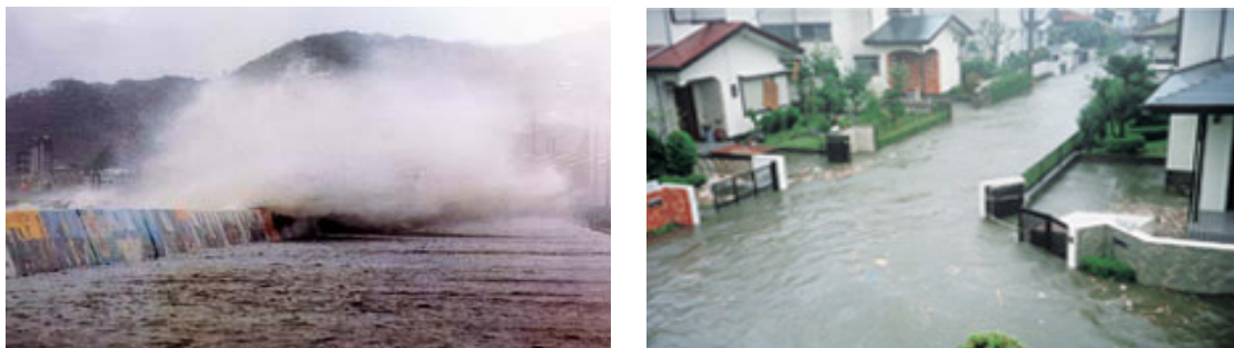
Fig. 10.1.1. Damage of Mahori coast
