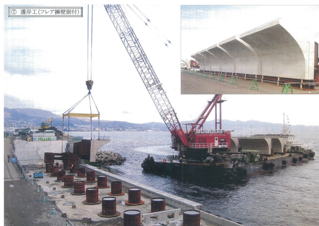
Fig. 10.1.10 Installation of Flare shore protection structure of Oita, Japan
