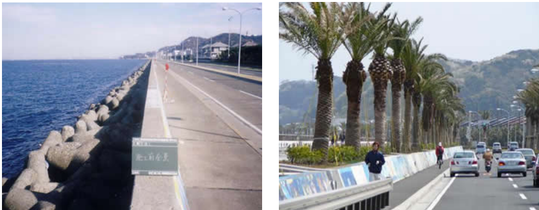
Fig. 10.1.4. Before and After of Coastal Improvement Project at Mahori coast
