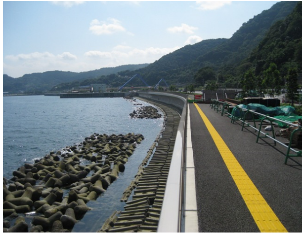
Fig. 10.1.12. Flare(Hybrid-type) Shore Protection using blocks
