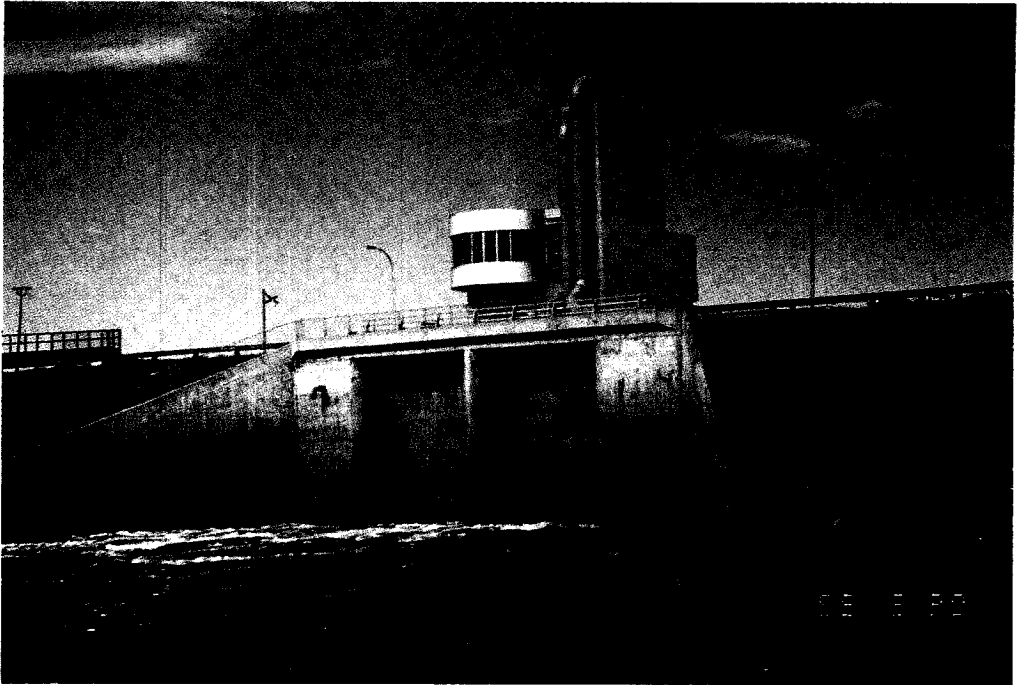
View from Downstream
