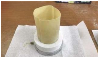
(e) Installation of shear rings
