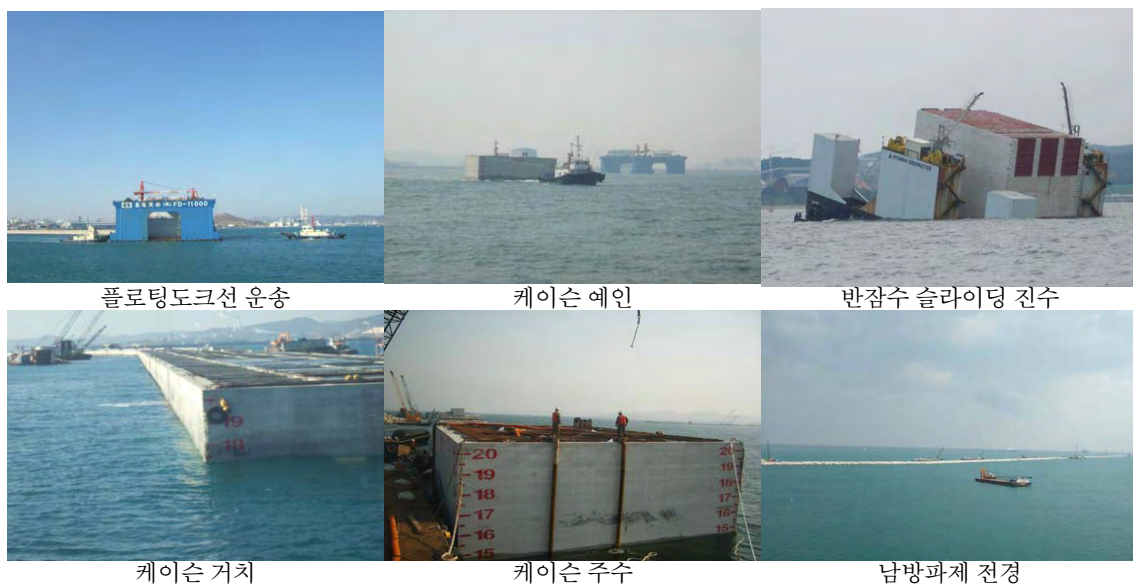
Fig. 1. Procedure in construction of caisson-type breakwater (울산지방해양수산청, 2004)
