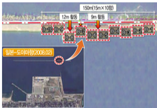
Fig. 1 Failures of Toyama Port
